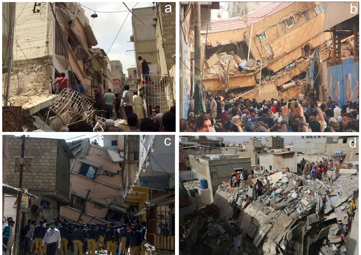
Figure 14. Land subsidence in different places of Karachi City. (a) Collapsed residential building at Rizvia Society, (b) Another collapsed at located in Soomro Street near Timber Market, Karachi City, (c) collapse residential building at Azizabad area, (d) Southern port city of Karachi.
