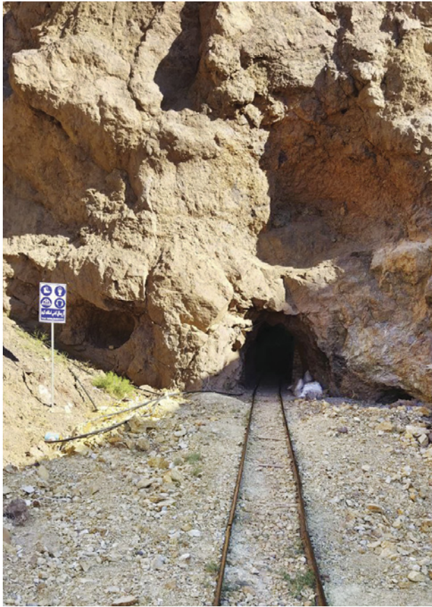
Figure 19. The Khoraj exploration tunnel is located in the south of the mine, and it is expected to join the mine's network below the Main tunnel. Photo by R. Farkhari.
